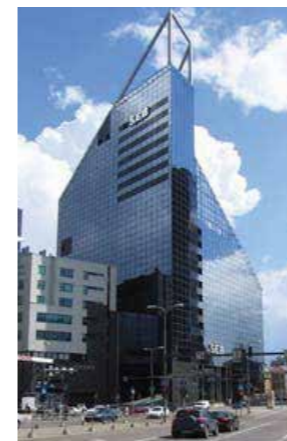
Estonia - SEB Building
